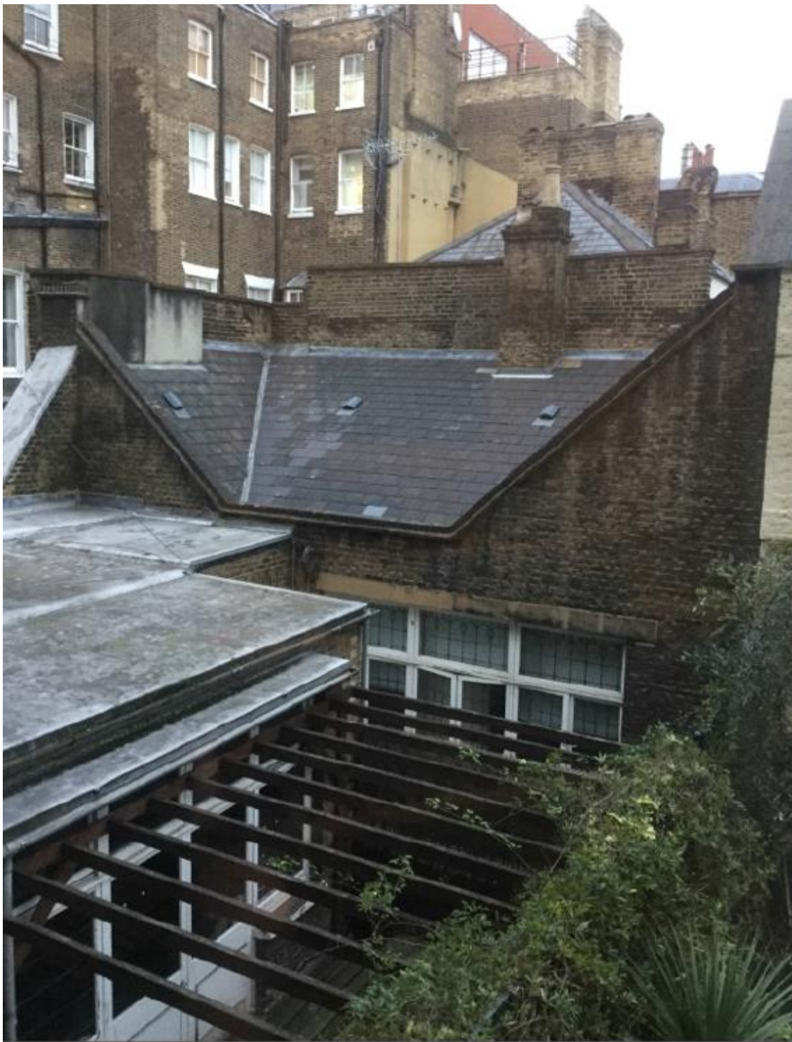
Outbuilding to rear:
